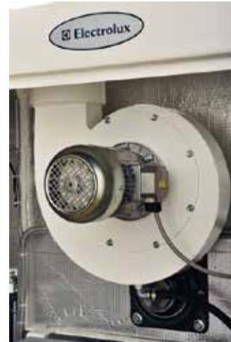
Most efficient dewatering on the market thanks to the large diameter off centred exhaust adjustable on each roll (not through the axis).
